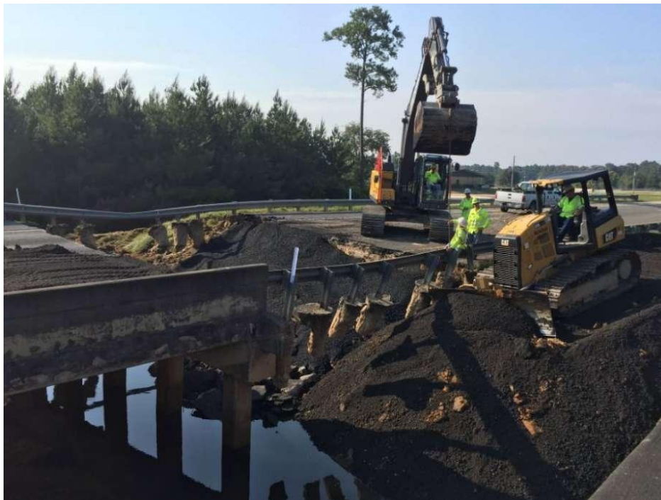
Fig. 11 Post hurricane road construction and repair activity on US96 at Village Creek near site 6
