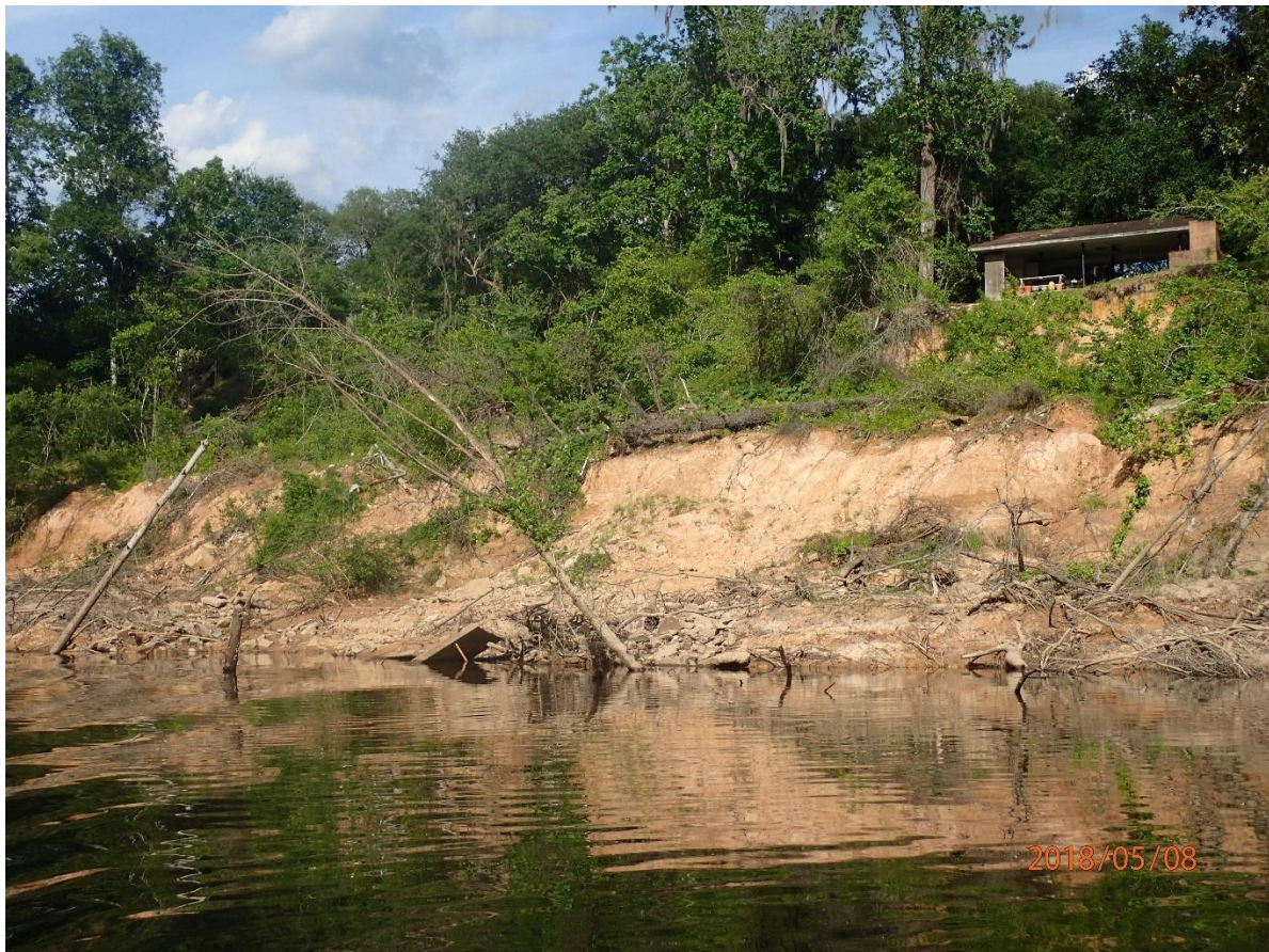
Fig. 8 Heavily eroded bank in the mid-reach of Village Creek, Hardin Co., Texas 2018.
